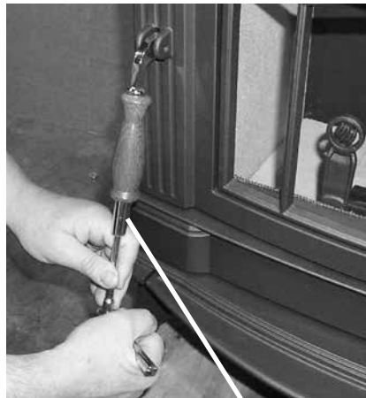
Secure using 7/16" socket wrench.
